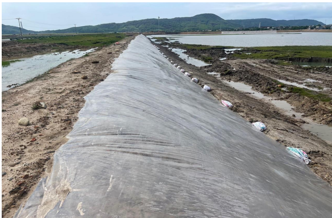
Figure 3.37 Containment area embankment and waterproof plastic liner
