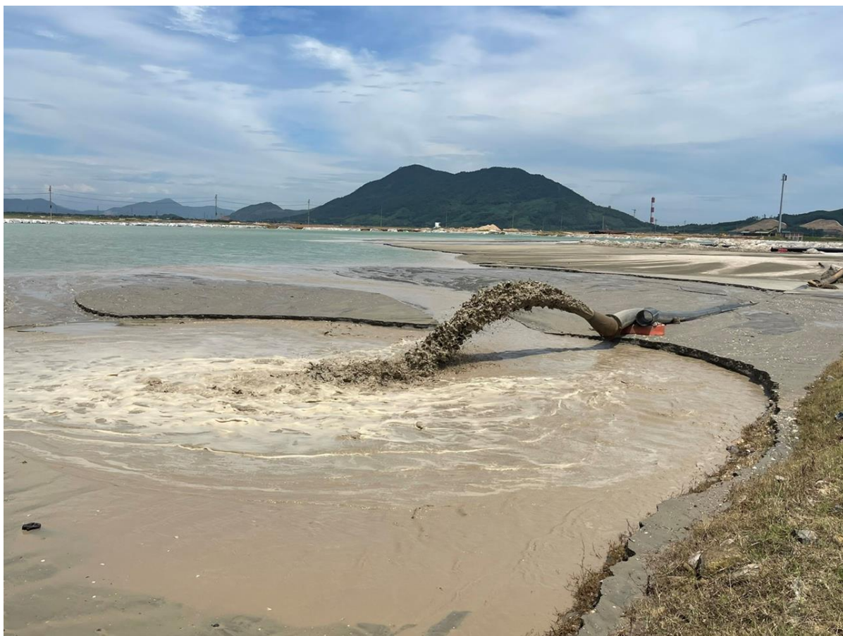
Figure 1.18 Pumping dredged material to storage area (actual image)
