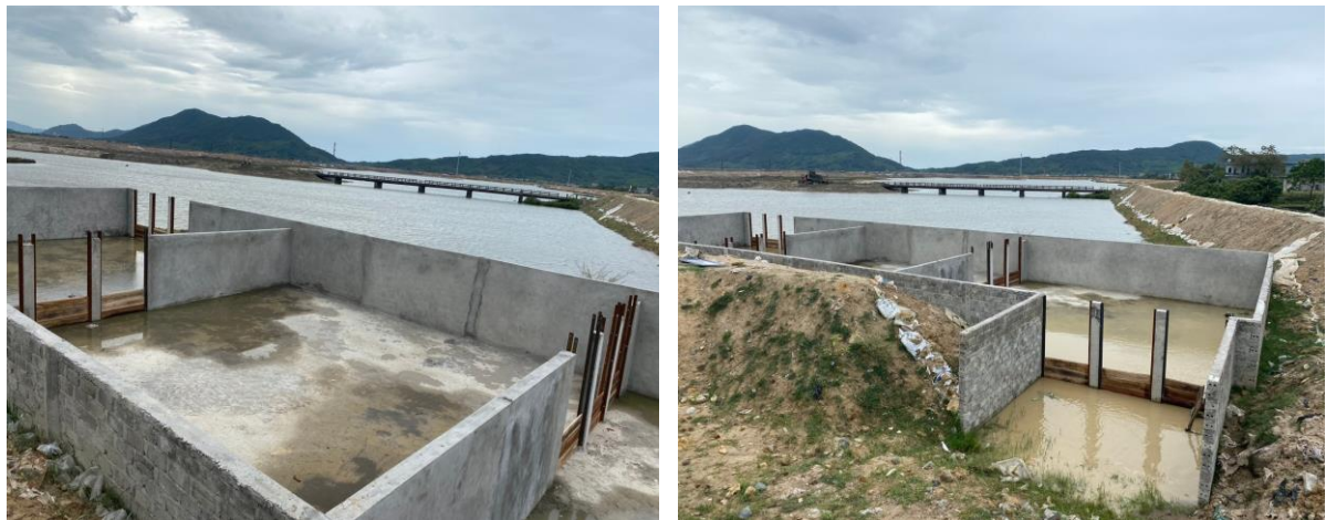
Figure 1.27 Three-compartment settling pond for treating runoff water from the storage yard.
