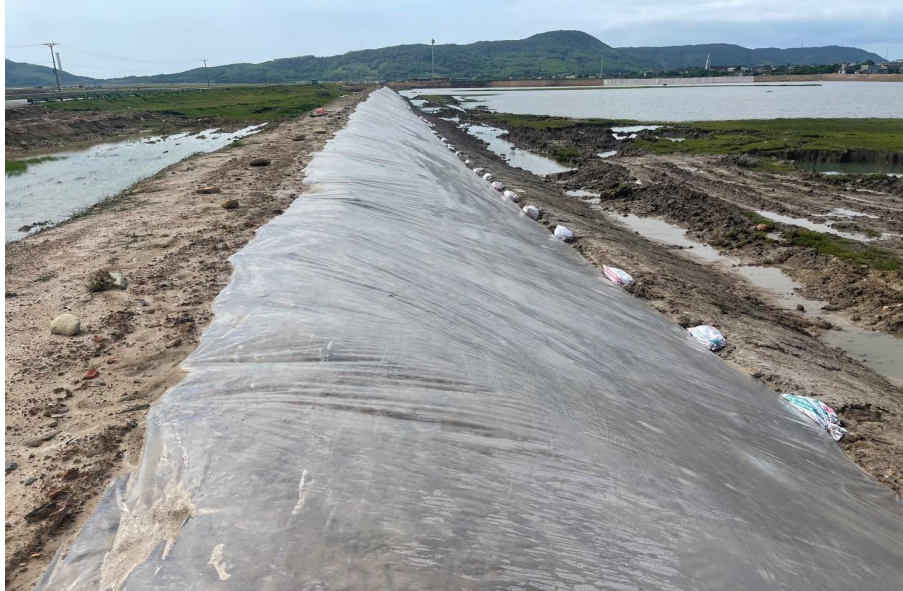
Figure 1.26. Embankment and impermeable nylon lining of the storage yard.
