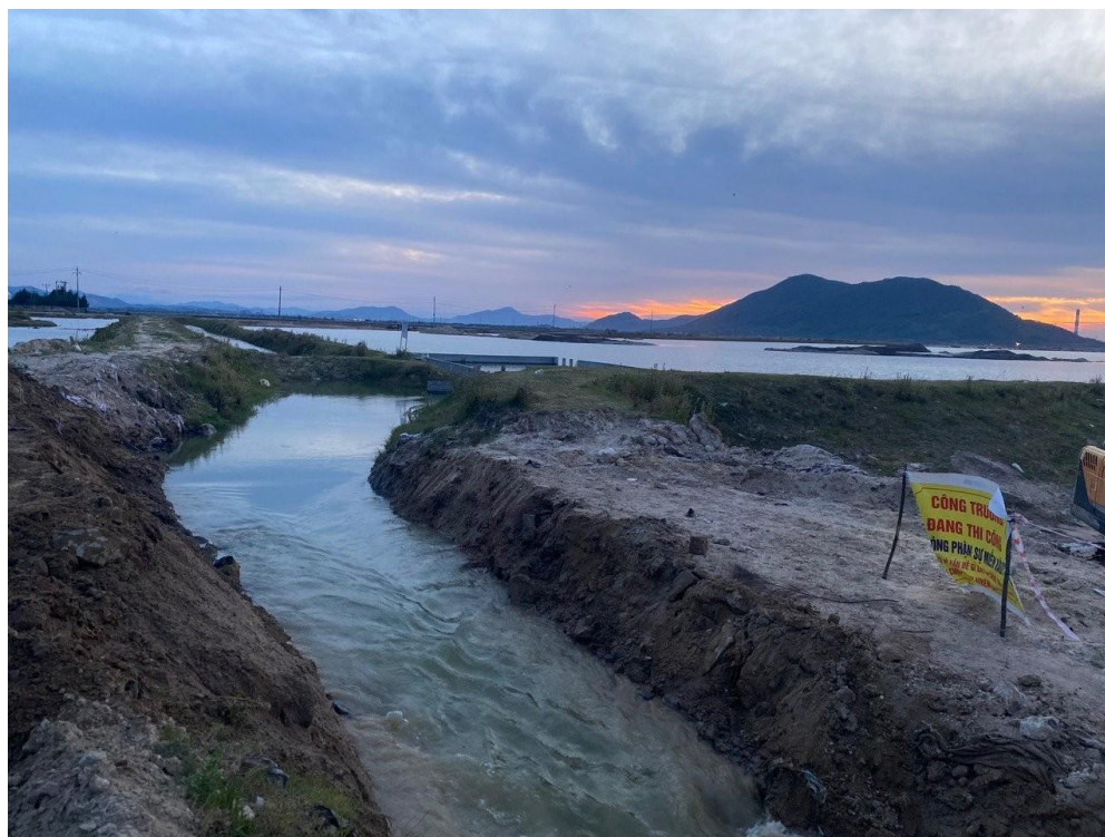
Figure 1.28 Open channel receiving water after the settling pond.
