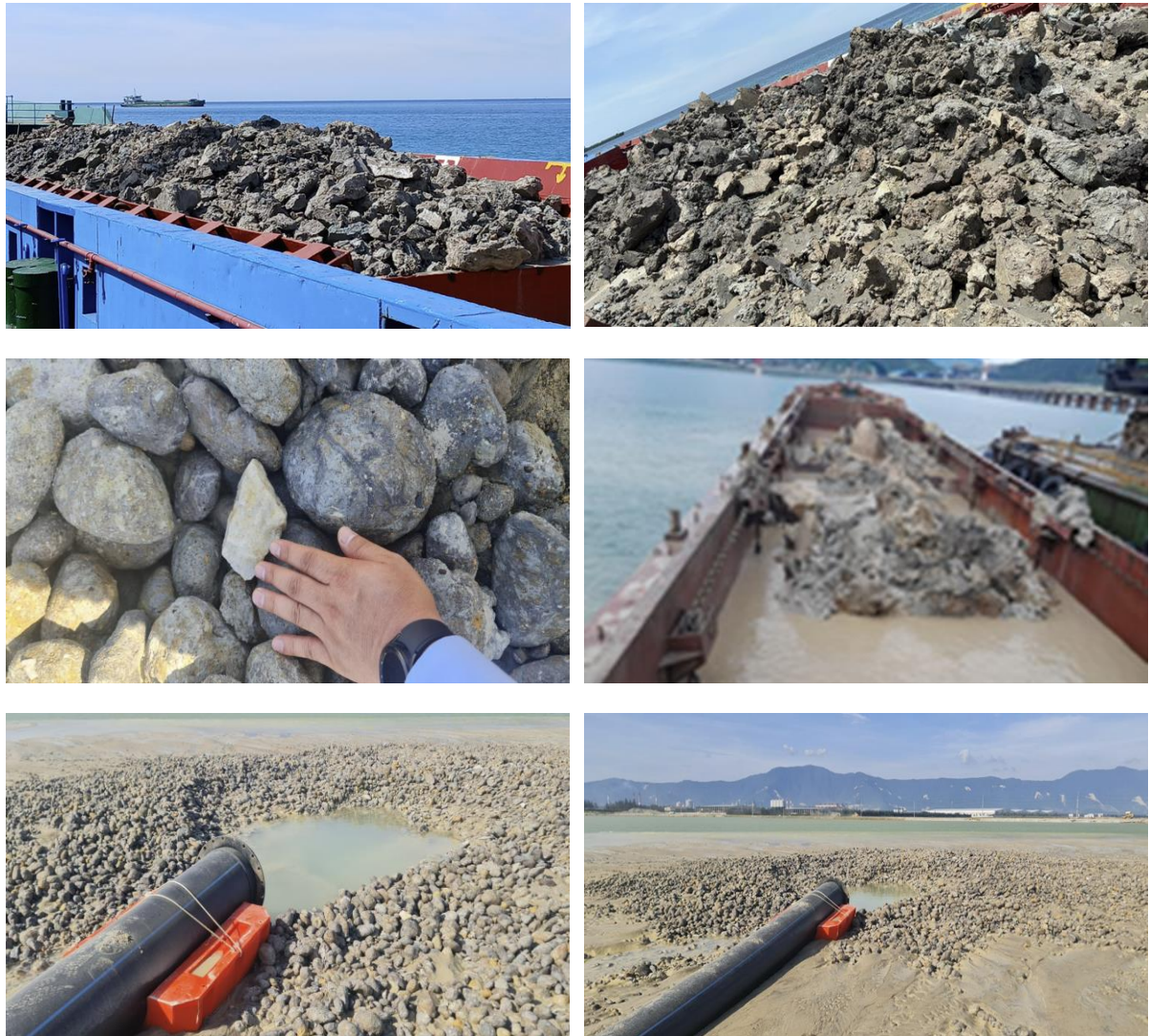
Figure 1.5 Some actual images of the dredged material after being loaded onto barges and pumped to the disposal site
