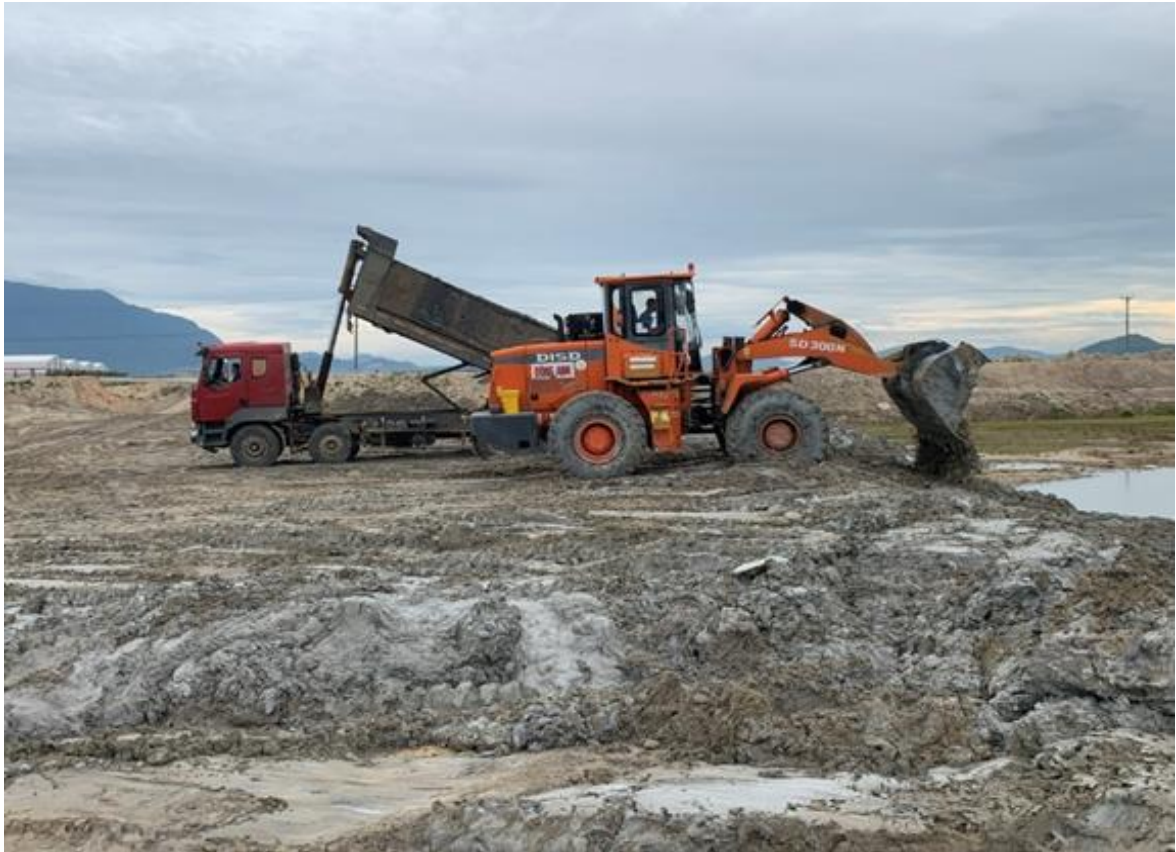
Figure 1.23. Illustration of the dredged material dumping and leveling process at the storage yard.
